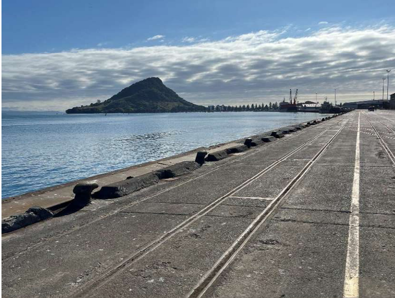
Figure 2. Example of a 'clean state' wharf apron and fender area
