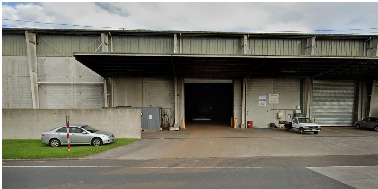
Figure 2 Main access doors onsite where discharges can occur (132 Totara Street)
