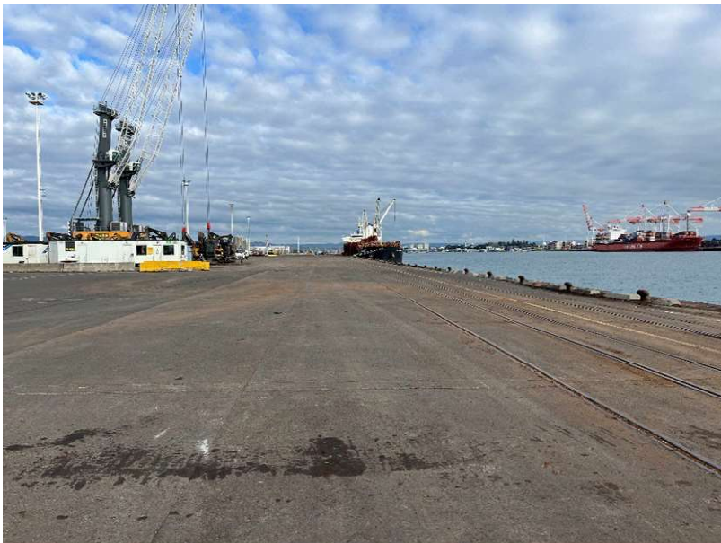
Figure 3. Example of a 'clean state' wharf apron
