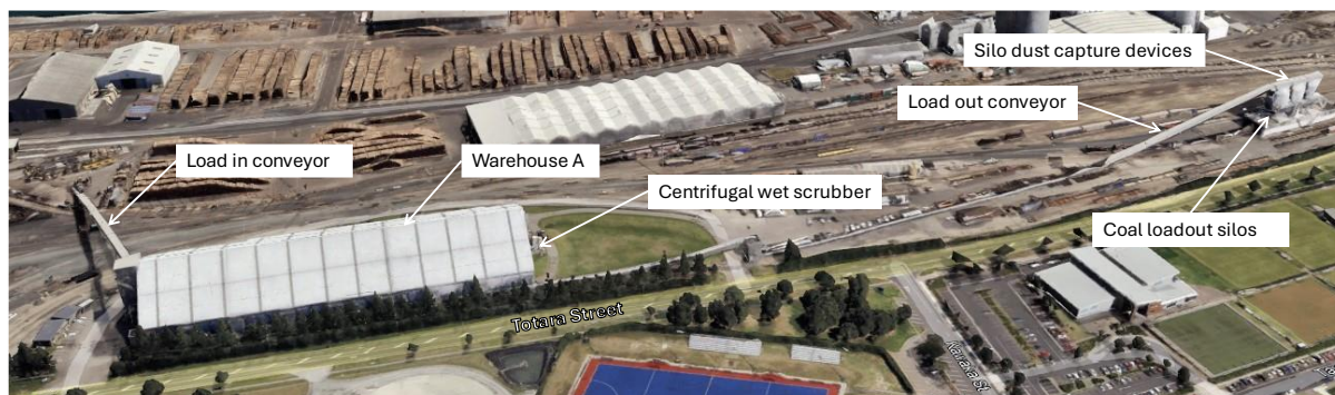
Figure 5.6: Location of Warehouse A – looking west (imagery sourced from Google Earth).
