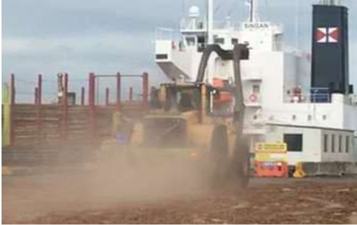
Figure 1: Example of excessive visible airborne dust
