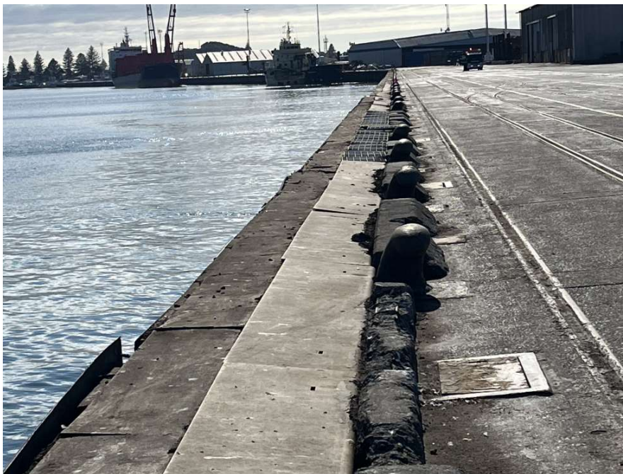
Figure 2. Example of a wharf edge in a 'clean state'
