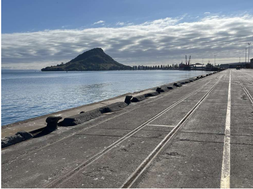
Figure 1. Example of a wharf apron in a 'clean state'
