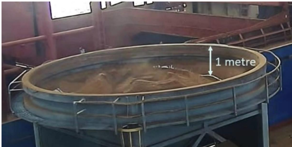
Figure 3. Maximum fill height of a hopper without a grizzly, hoppers A and B
