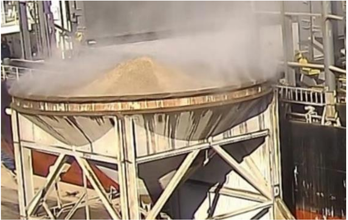
Figure 4. Maximum fill height of a hopper with a grizzly, hoppers C to J
