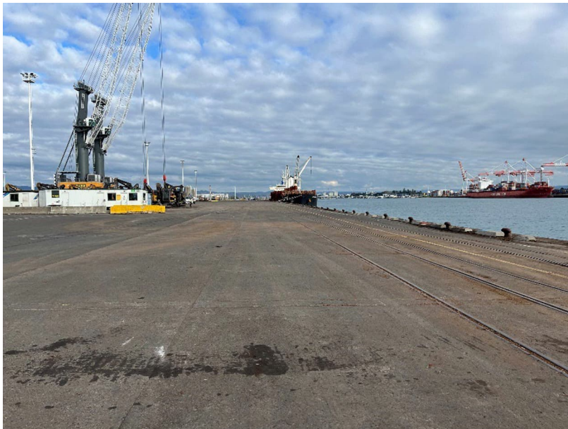
Figure 3. Example of a 'clean state' wharf apron
