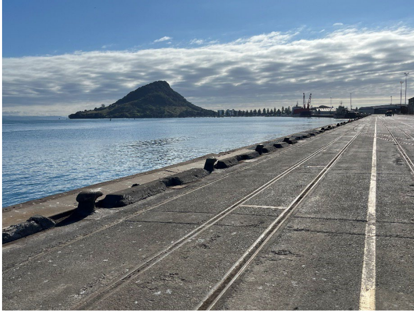
Figure 1. Example of a 'clean state' wharf apron and fender area
