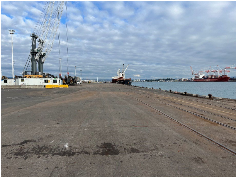
Figure 2. Example of a 'clean state' wharf apron
