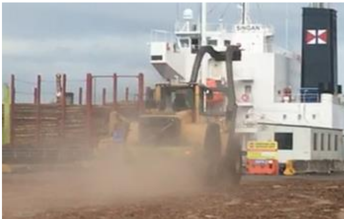
Figure 1. Example of excessive visible airborne dust.
