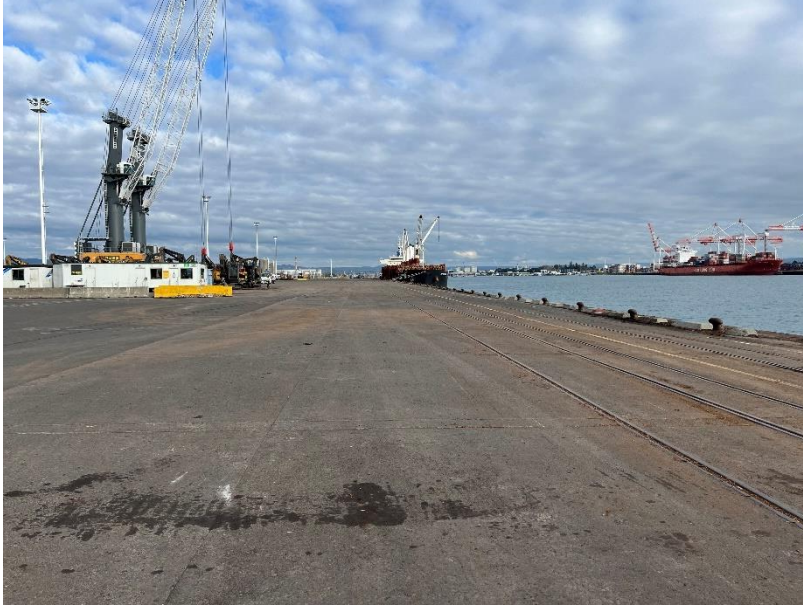
Figure 3. Example of a 'clean state' wharf apron
